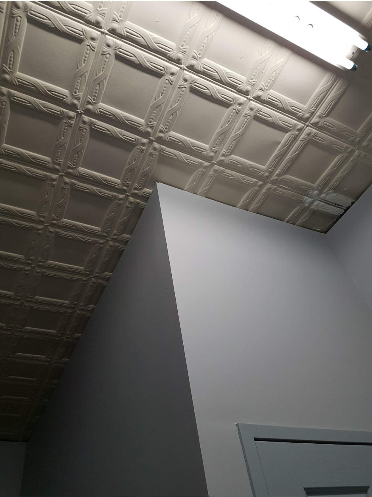
Internal view. A stud wall rises directly to obscure the original decorative ceiling. Modern Fluorescent Lighting fixtures have been installed insensitively over the original ceiling
