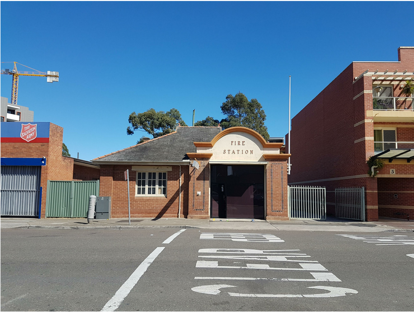
Eastern Facade. View of the Heritage Fire Station building from William Street. The front facade is dry pressed face brick with a dark brick feature panel either side of the original garage door opening. An Arched feature parapet spans above the original Garage door opening. The Dutch Gable roof is Slate with terra-cotta hip and ridge tiles, and terra-cotta finials.
