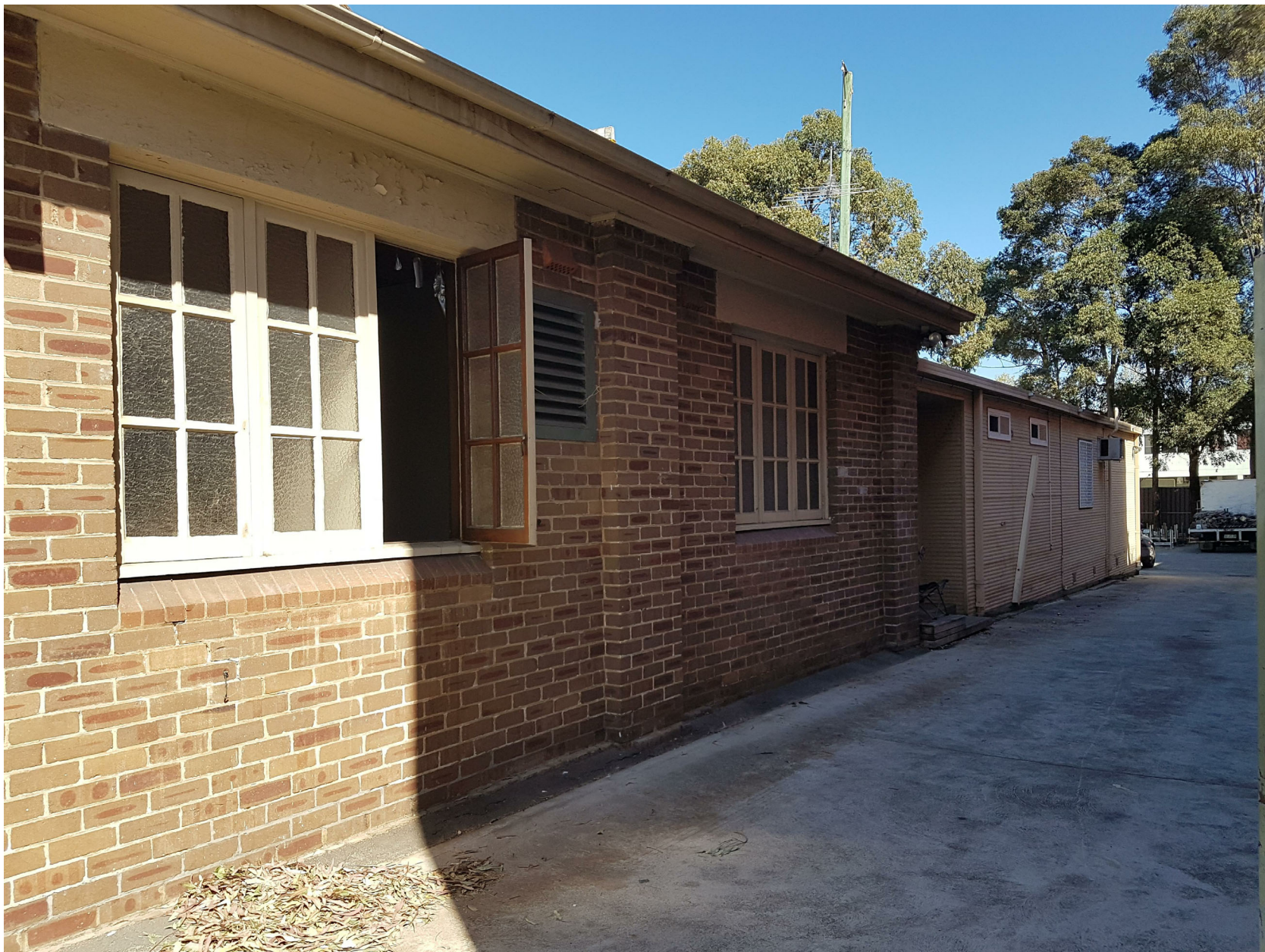
Northern Facade. The original fabric is common brick with Timber framed Casement windows. A weatherboard prefabricated extension extends to the rear (West).
