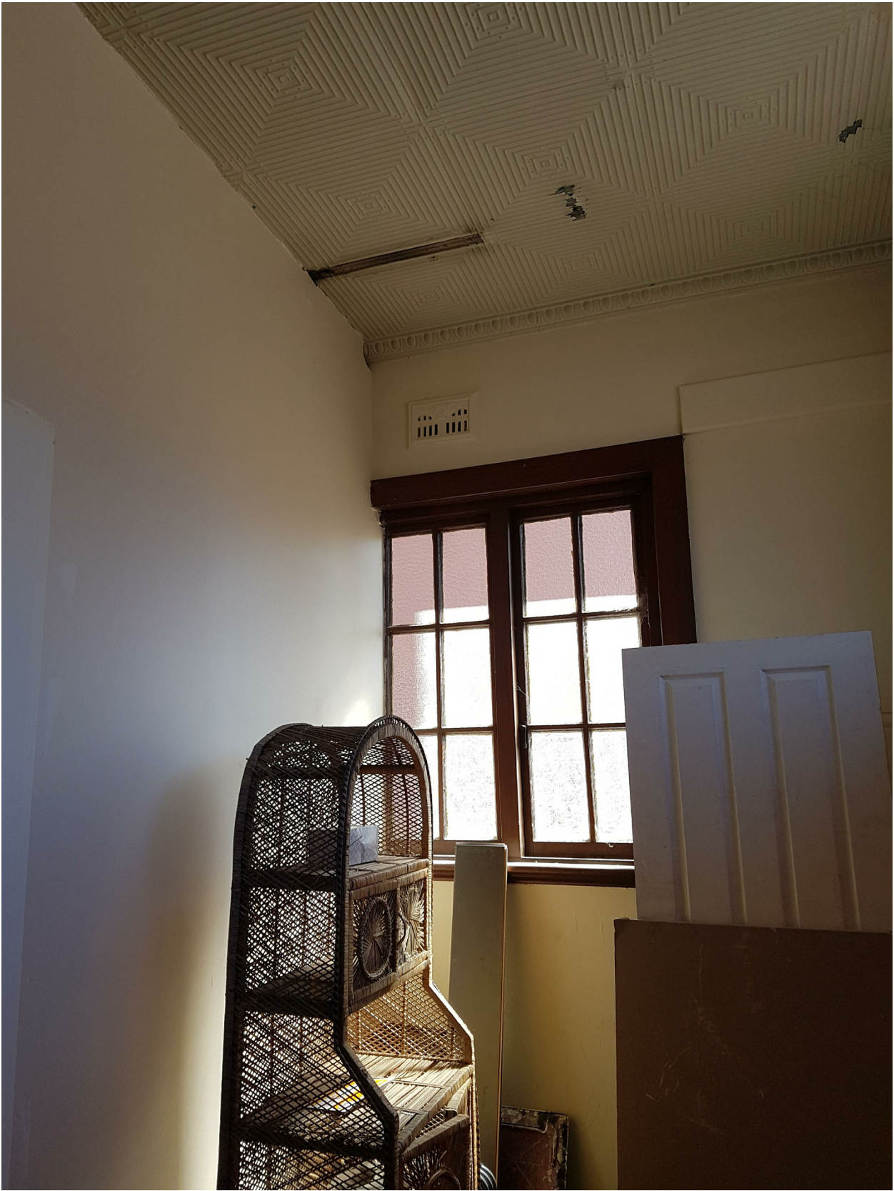
Internal view. A stud wall added for the extension interrupts an original triple panel timber casement window. The original ceiling appears to have been damaged.
